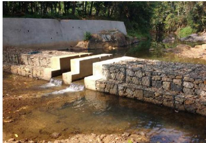
*Figure 4. Gabion Check Dam*
